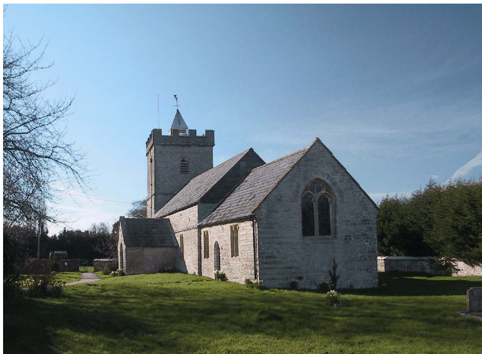
St. Peter's Church, viewed from the east
